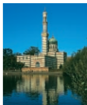
The steam engine house as a "mosque" on an inlet of the Havel
