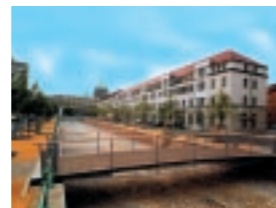
The rebuilt Stadtkanal
